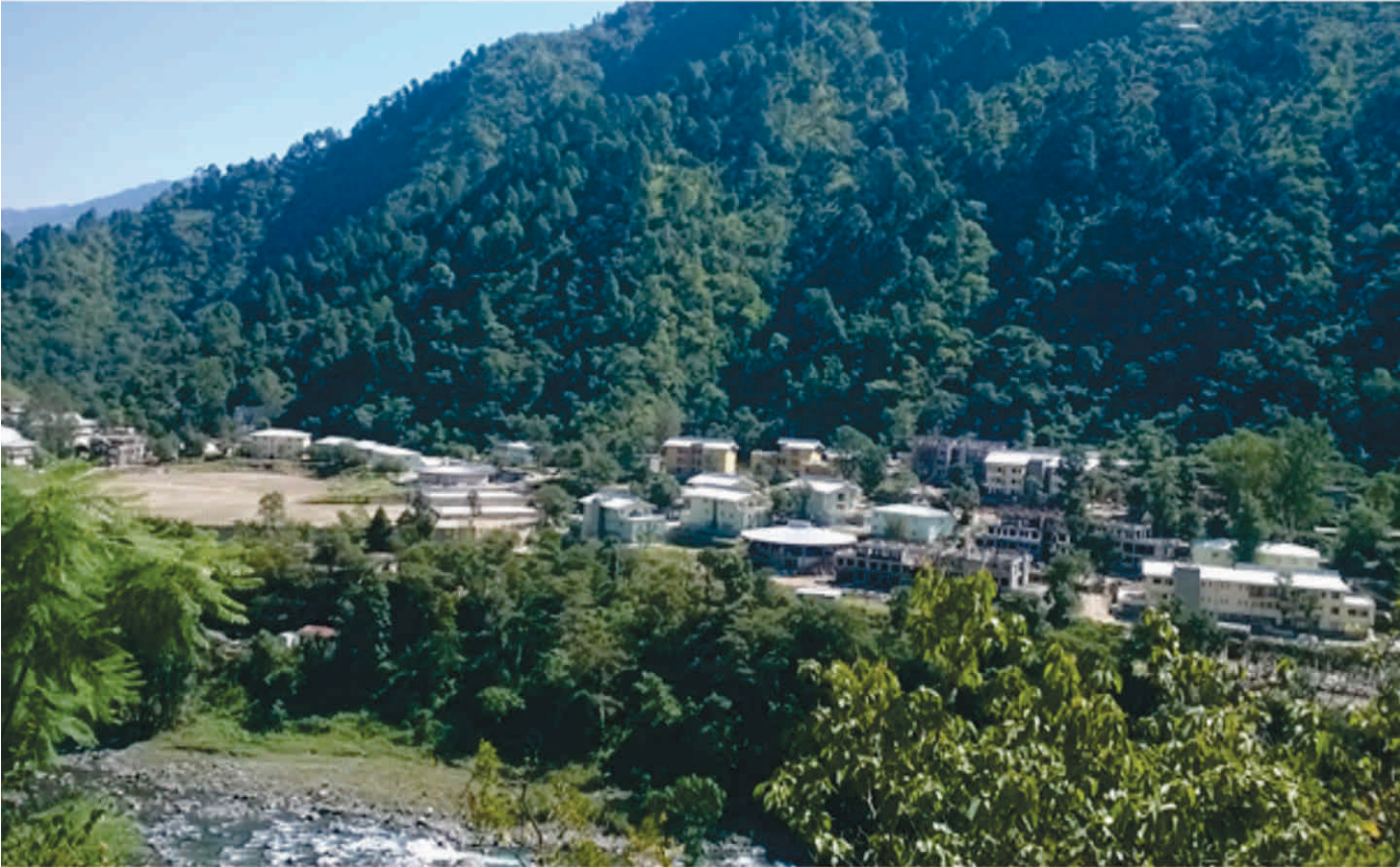
Buildings Already Constructed and Work in Progress (South Campus)
