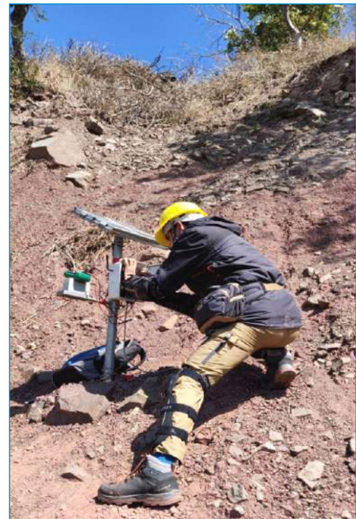
Team member installing system on a landslide
