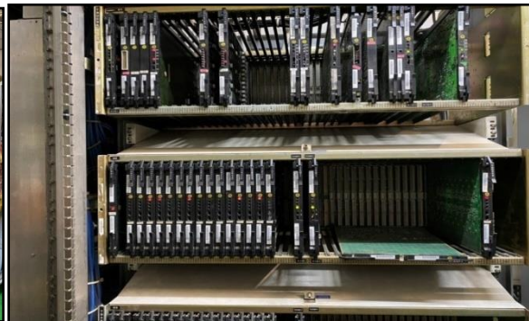
Switch Panel: Server Room Telephone Exchange: Line Cards
