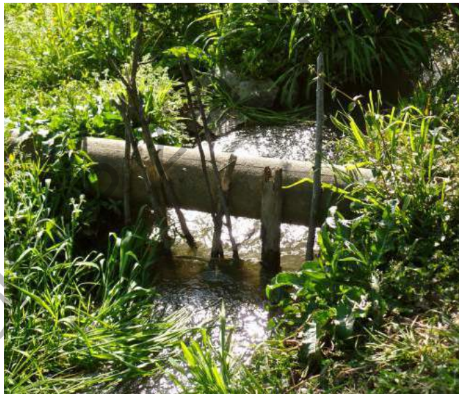
Figure 3. Common canal filter comprised of vertical sticks.
