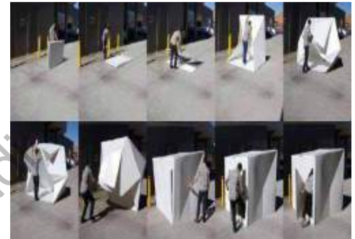
Figure 9. Pryor's polypropylene emergency shelter.
