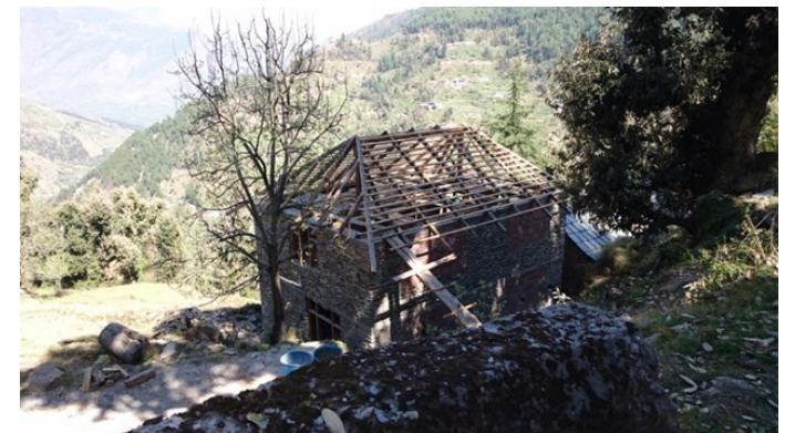
Figure 1.3-House built using Bamboo Retrofitting
