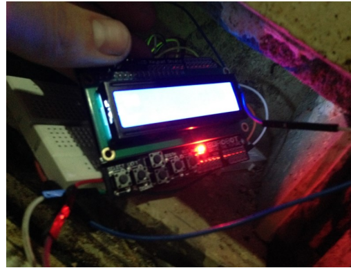
Figure 6: Additional electronics and LCD screen for tray counter
