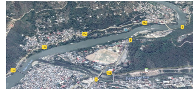
Figure 5. Map View of National Highway 154 (left side Beas River) and National Highway 3 (right side of Beas River) through the middle of Mandi town and crossing the Suketi Khad River)
