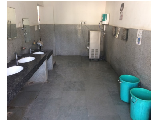
Figure 3: The waste disposal area at D2 mess
